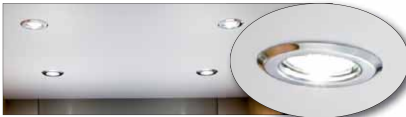
Ceiling with halogen spots
