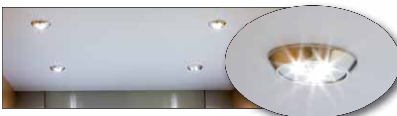
Ceiling with LED spots
